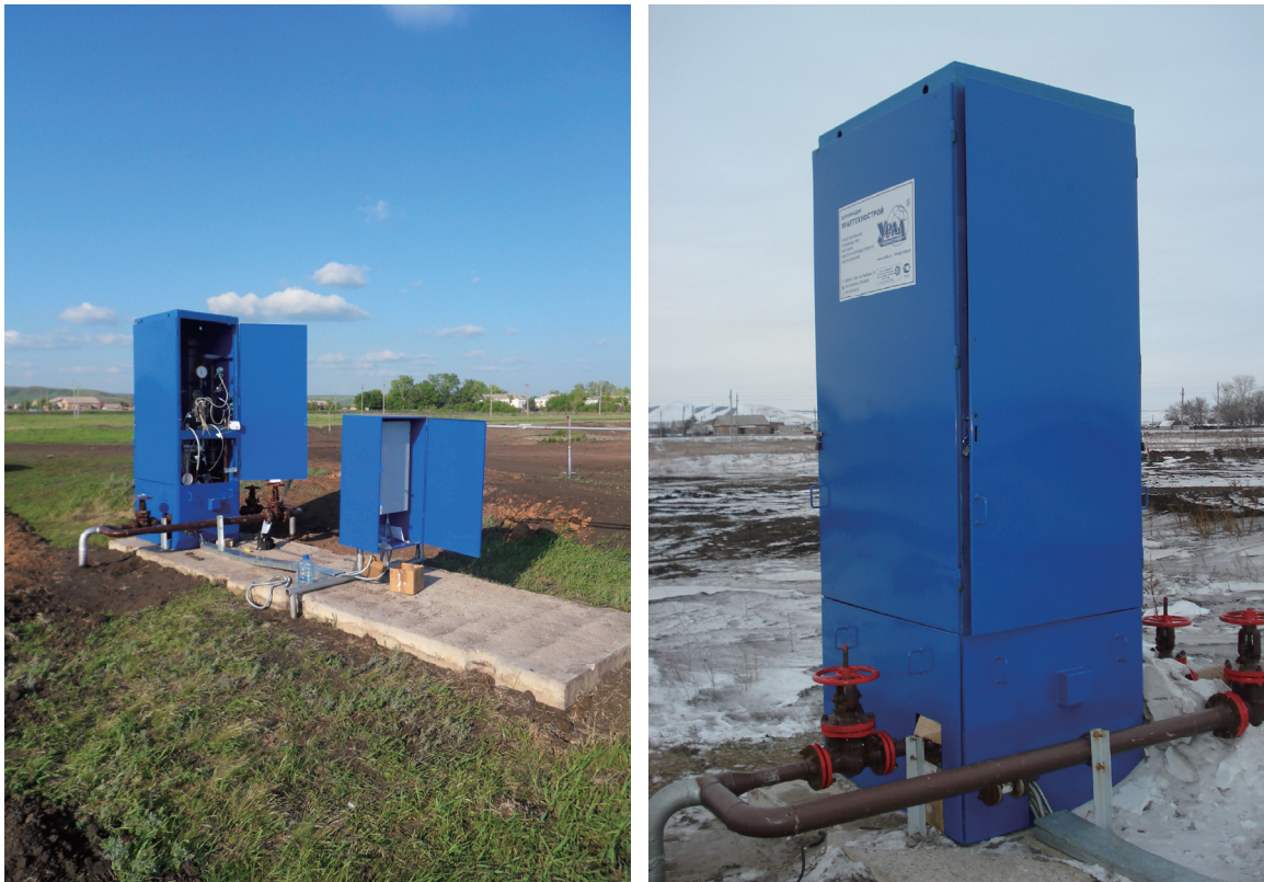
Figure 2 The General View MPD of Which During the Field Testing
